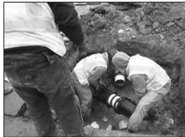
City workers Bobby Carpenter and Joey Courtney manhandling a new section of pipe and couplers into position at the location of the sewer line break in Windward Slopes on New Year's Eve. Supervisor James Stimpson has his back to the camera.
