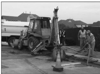
City workers Bobby Carpenter and Joey Courtney manhandling a new section of pipe and couplers into position at the location of the sewer line break in Windward Slopes on New Year's Eve. Supervisor James Stimpson has his back to the camera.
